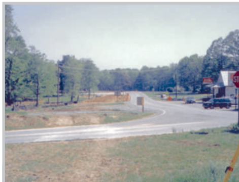
This simplified intersection in Volens now has much-improved sight distance.
