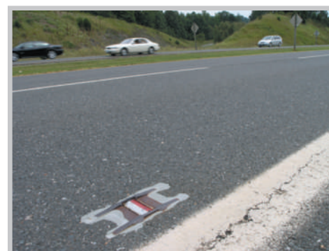
Hundreds of reflectors have been imbedded in 501's pavement around Lynchburg.
